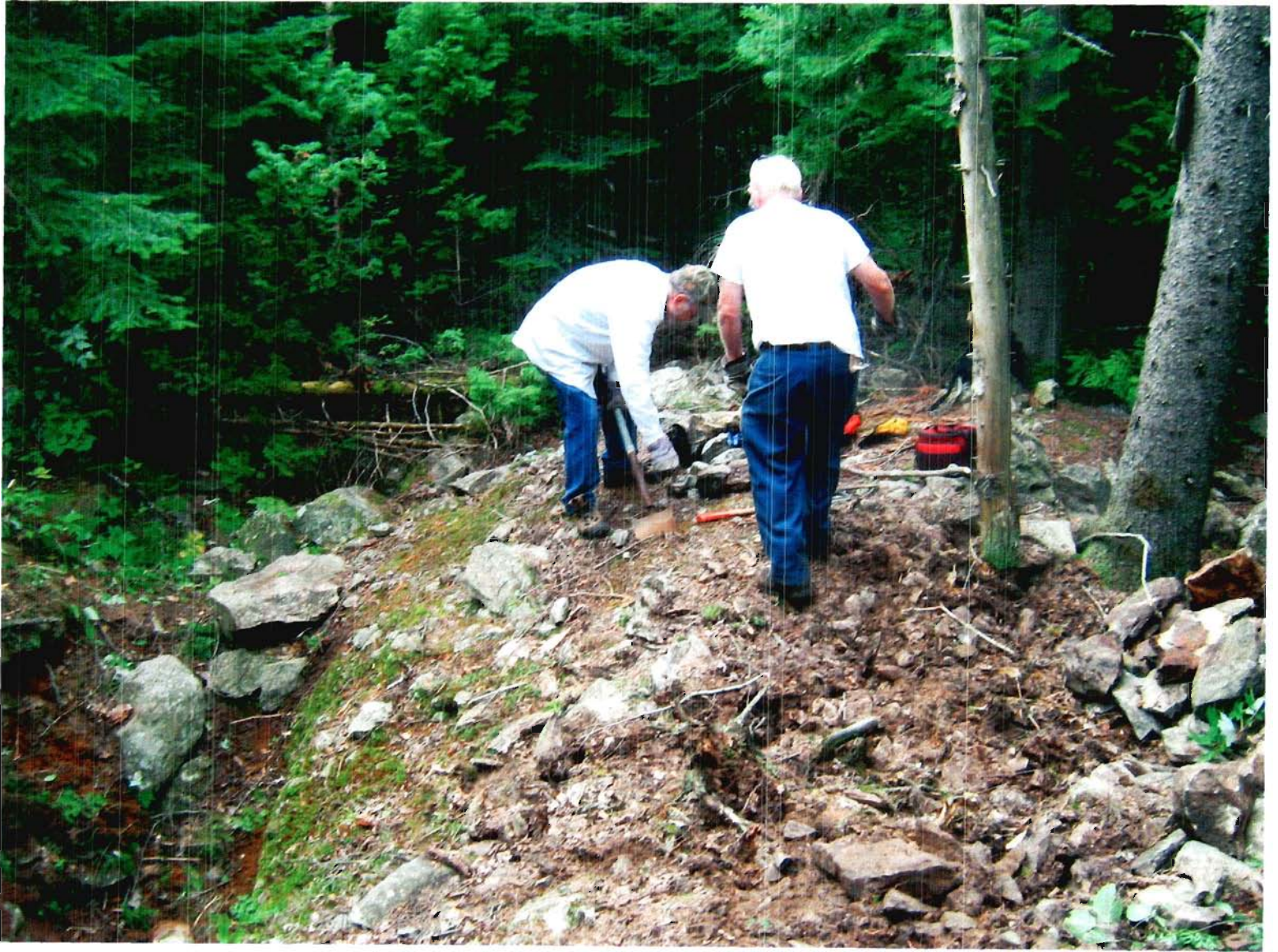
SOUTH WEST END OF TRENCH
