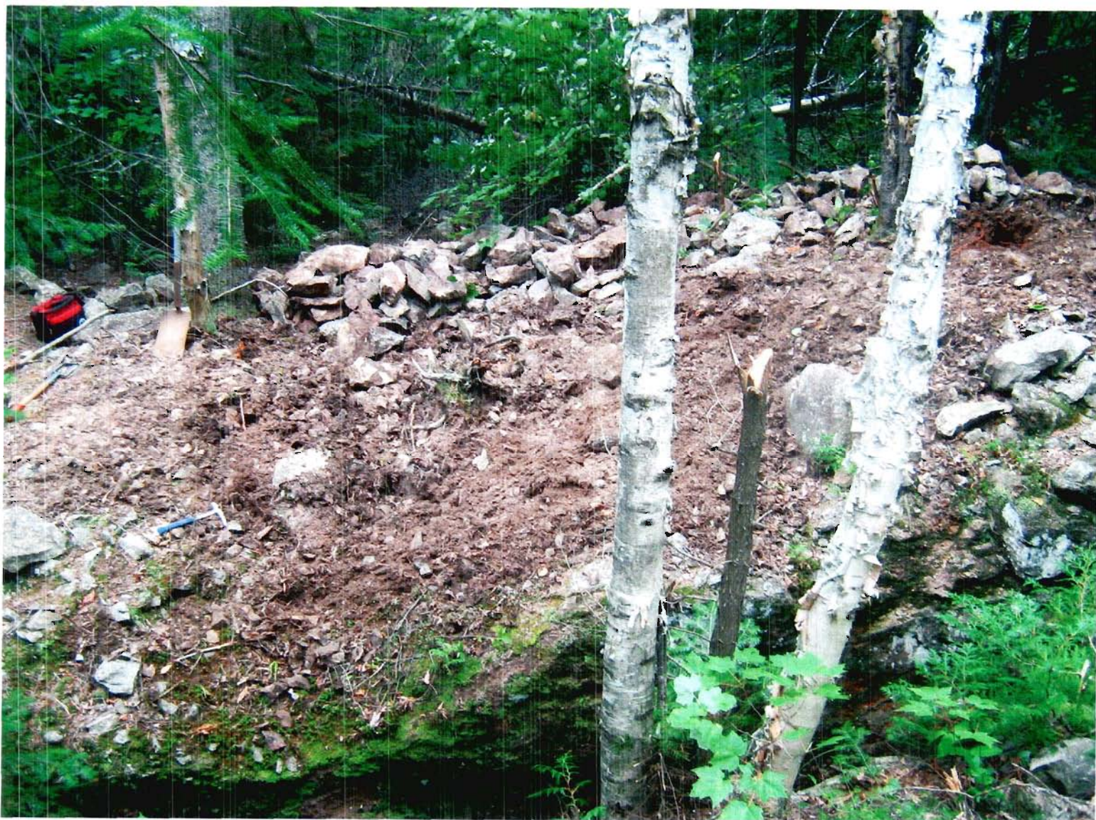
SOUTH WEST SIDE OF TRENCH
