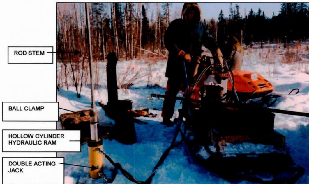
FIGURE 7 OVERBURDEN DRILLING; ROD JACKING OPERATION
