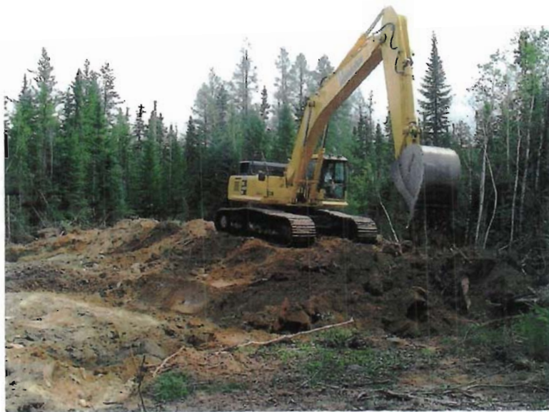
PICTURE 1 SHOVEL ON NORTH PART OF TRENCH
