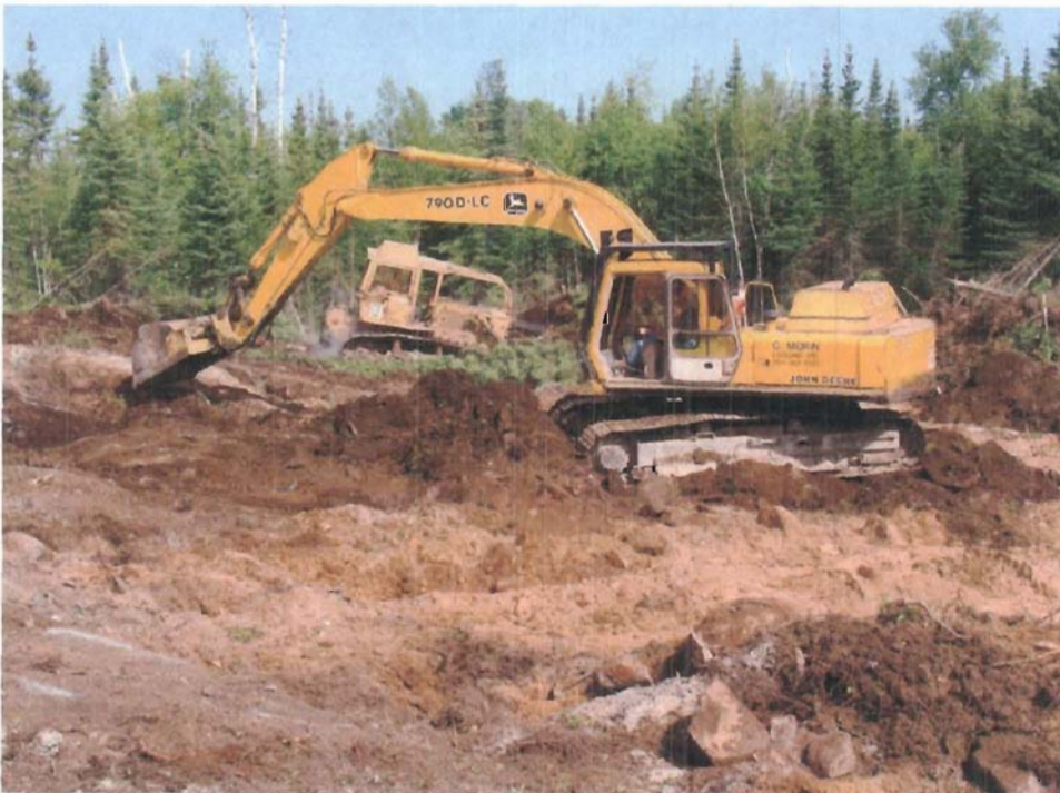
Photo 2. – Stripping with backhoe and dozer
