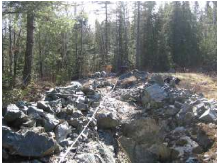
Figure 3: Previously Blasted Trench A (Photo taken, April 2007).
