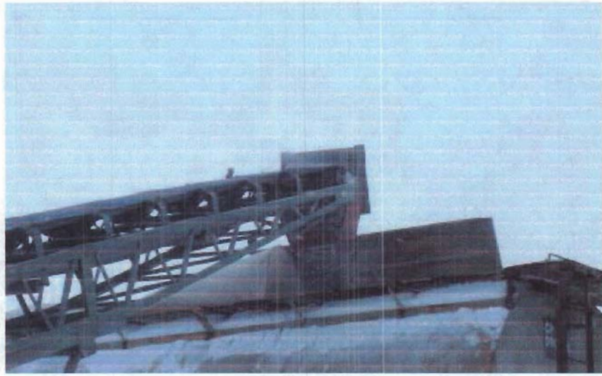
Photo 5 – Loading of Ore into Rail Car
