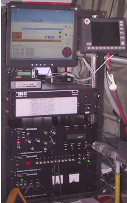
Figure 7. AeroTEM II Instrument Rack., including AeroDAS and RMS DGR-33 systems, AeroTEM power supply, data acquisition computer and AG-NAV2 navigation system.
