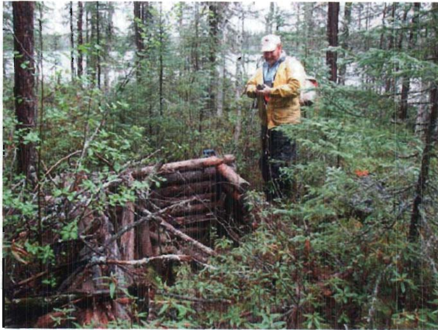
Figure 12. Structure 4. Remains of a small building. Looking east.
