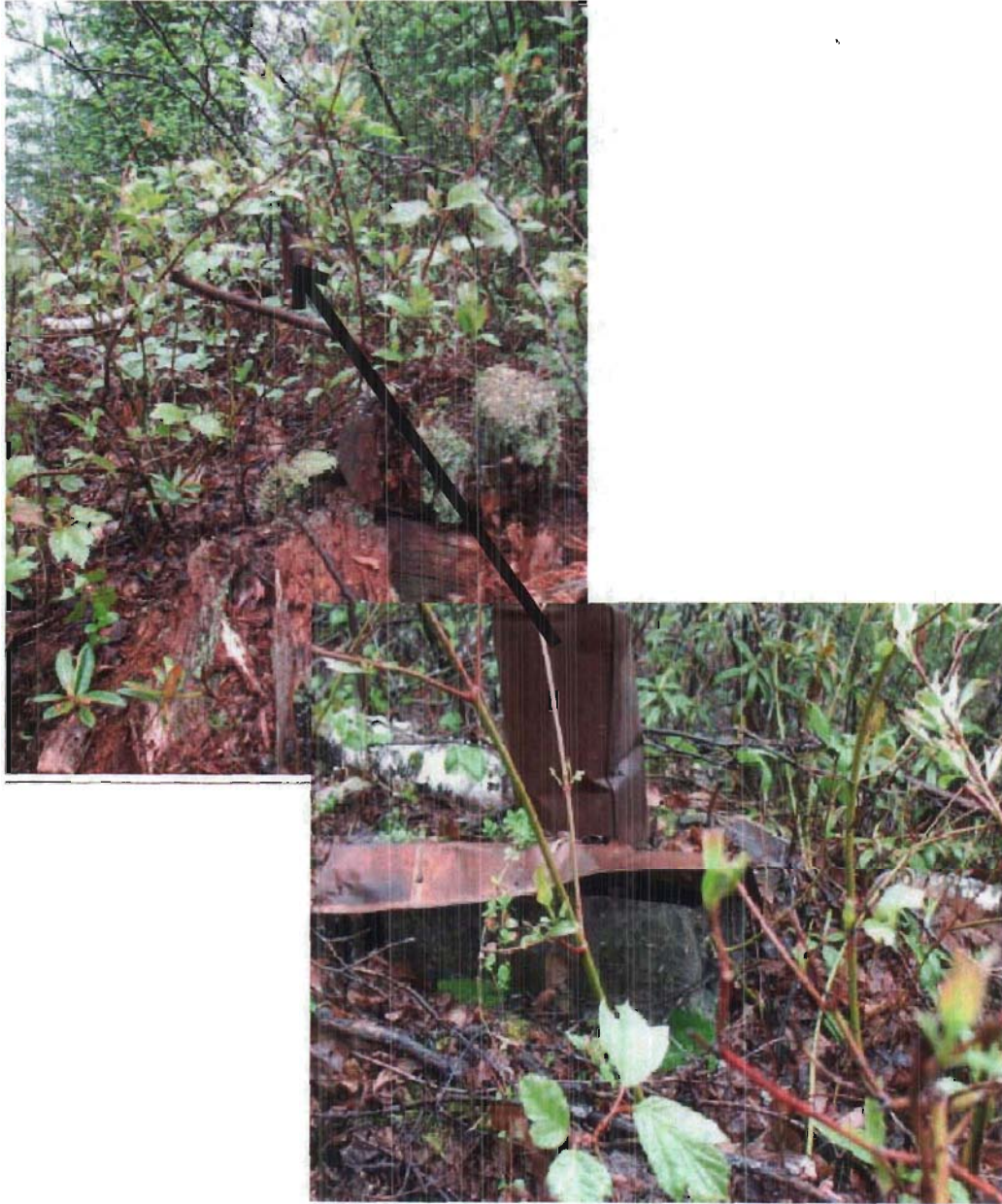
Figure 9. South wall of structure 1 (top photo). Looking west. Chimney and cement base on south wall (bottom photo). Looking north.
