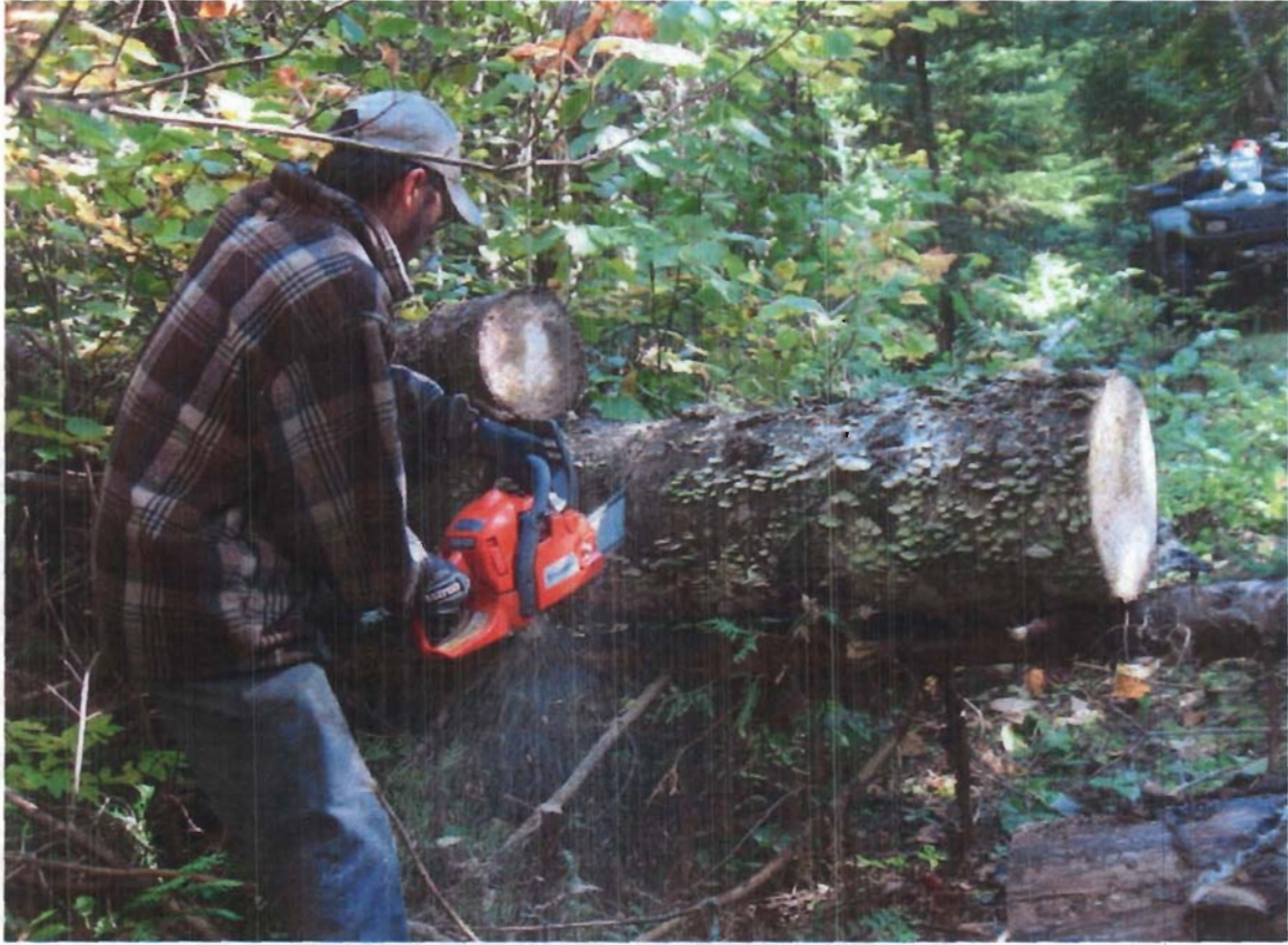
Pole Lake Access Trail Construction
