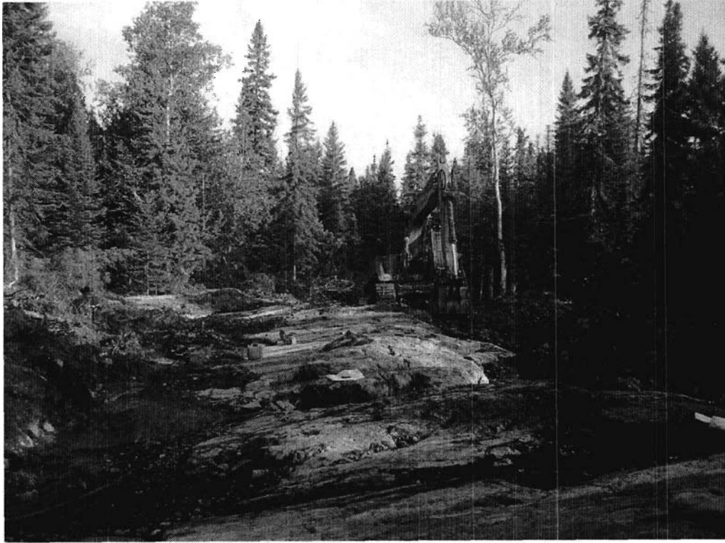
Cat 235 Excavator in Trench A.
