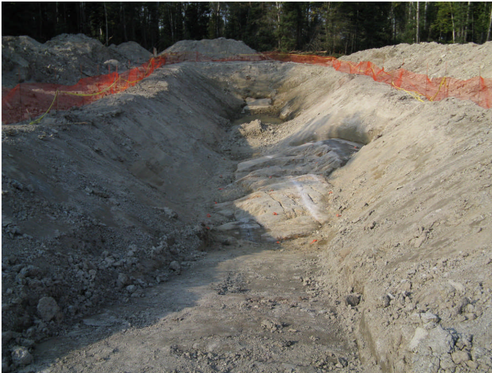
Figure 9-1-Trench # 1, Goliath project, Ontario.
