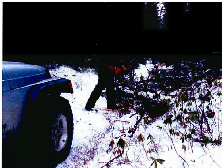
Re-cutting old road - November 21, 2010
