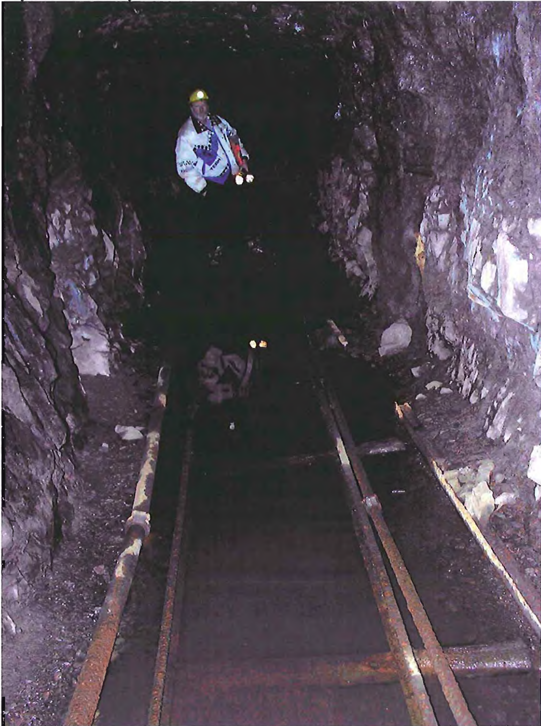
Photo 1: D. Currah, Sarissa consultant, inside the Adit – shows the condition after 50 years of inactivity.
