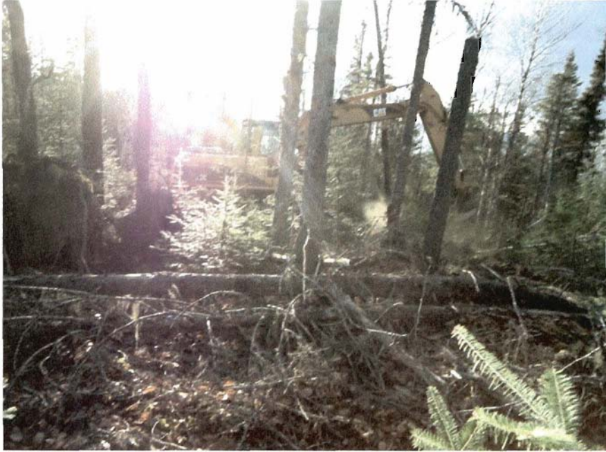
Pic 9- Trenching on Claim # 4265718
