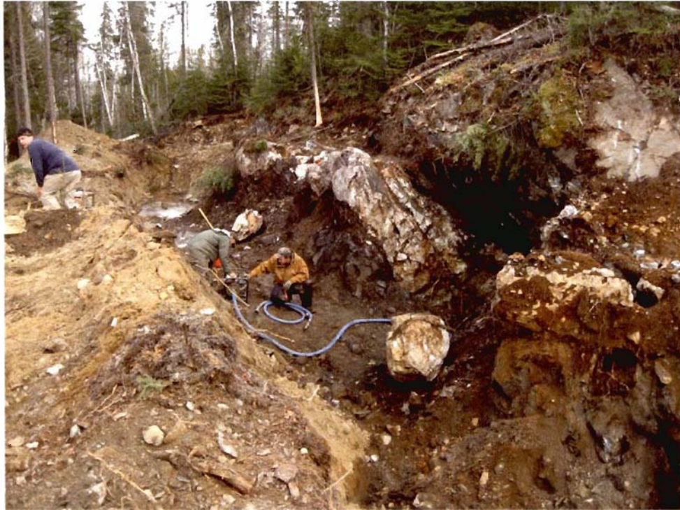
Opening up and preparing for channeling of the main Bucksaw Vein Trench #1 Area
