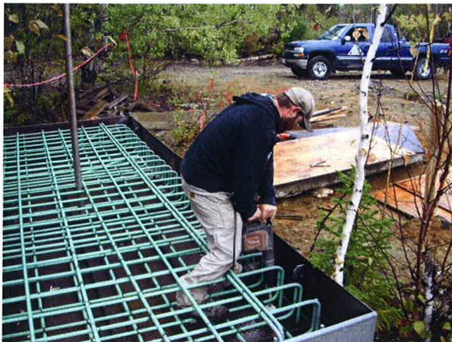
4. Cap dowel installation being completed.
