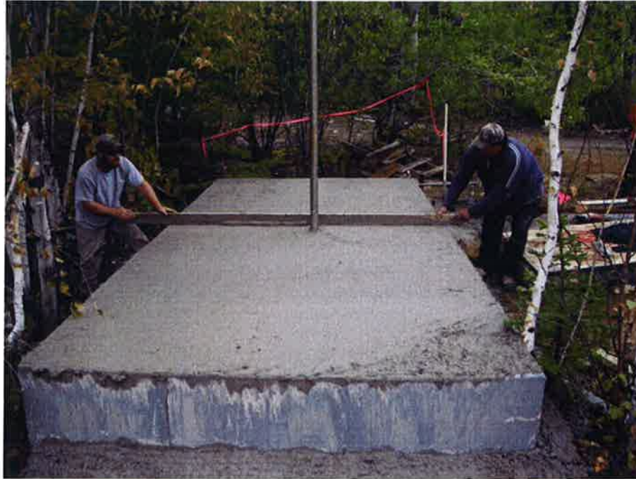
5. Concrete pour and surface finishing is completed.
