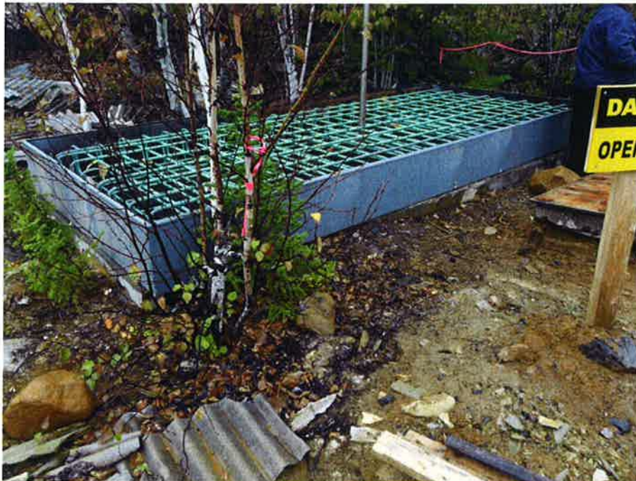
3. View of formwork and rebar prior to pour.
