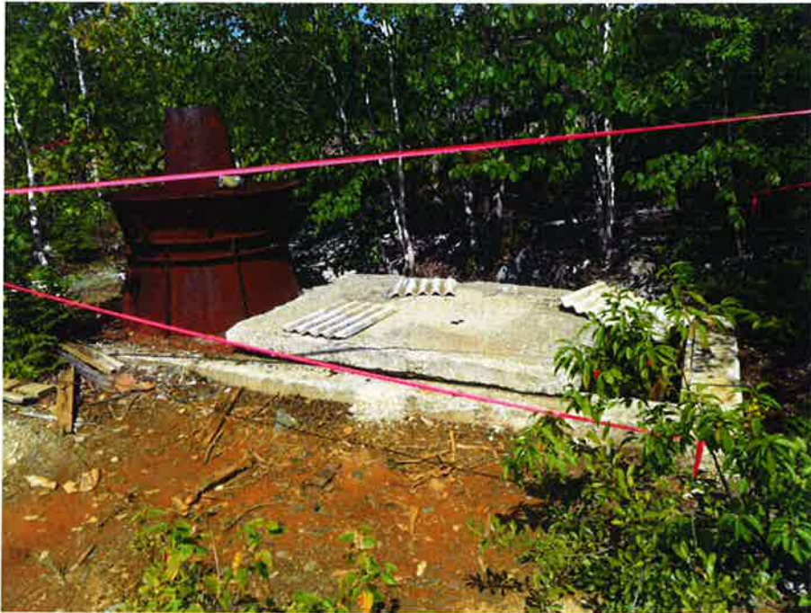
1. View of original shaft looking north.
