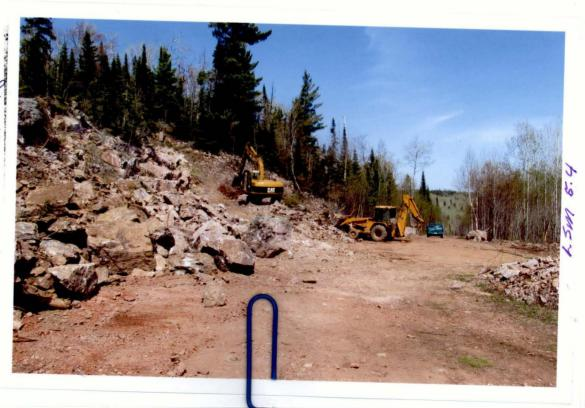
LSM 5.5 TUESDAY MAY 28-2013 THIS PICTURE SHOWS THE EXCAVATOR STRIPPING THE MID-POINT AREA OF THE SOUTH SLOPE, PILING IT FOR THE BACK HOE
