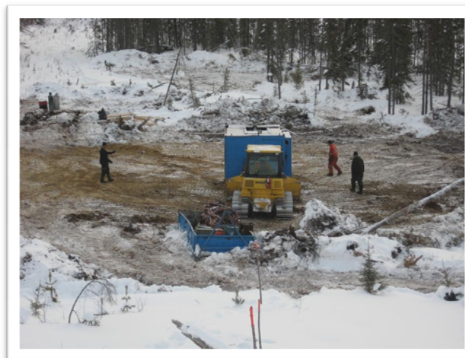
Figure 4: Positioning the drill onto the setup for CO-10-002 (photo).
