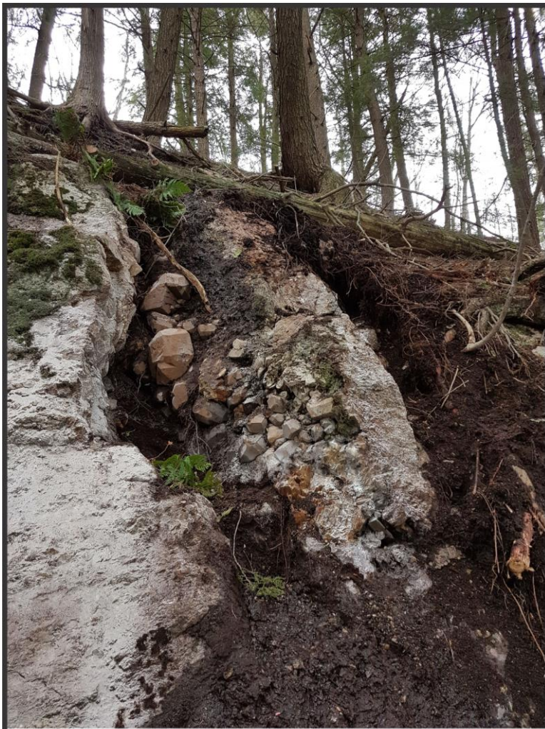
Figure 7; Photo showing fissure after some wall rock was removed.
