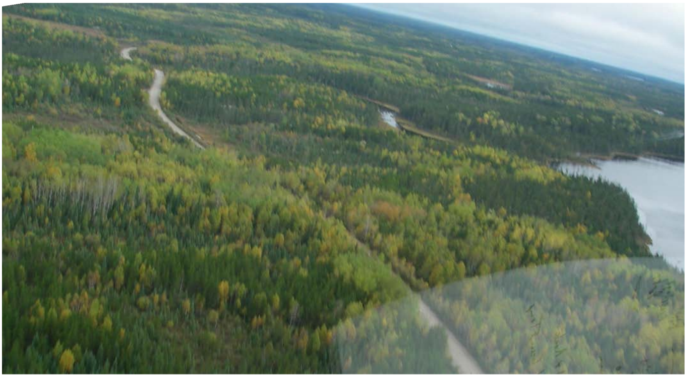
VIEW LOOKING NORTHWARD AT STATION 23+000 SHOWING ADJACENT ACCESS ROAD AND TYPICAL SPRUCE-BIRCH FOREST OVER SHALLOW BEDROCK.
