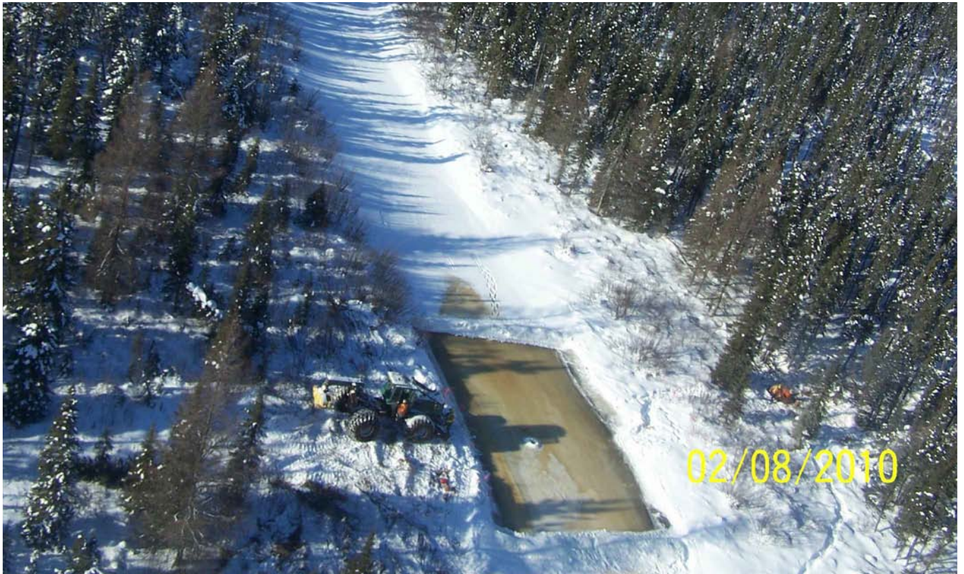
ICE PAD CONSTRUCTION AT SMALL RIVER CROSSING ALONG SOUTHERN SEGMENT OF CORRIDOR.
