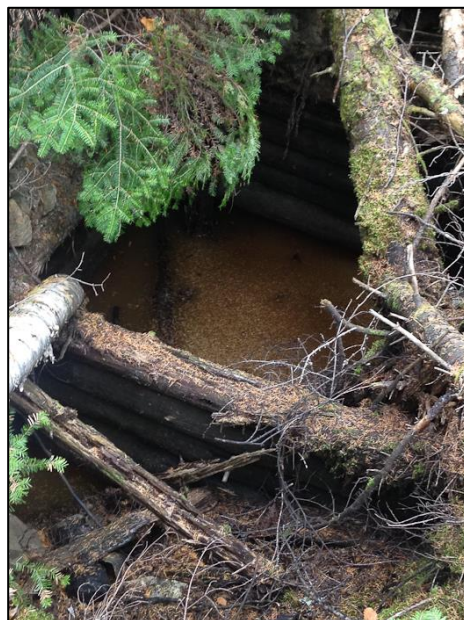
Photos: Kirgood Shaft with steep sides - recommended to fence off hazard (below)
