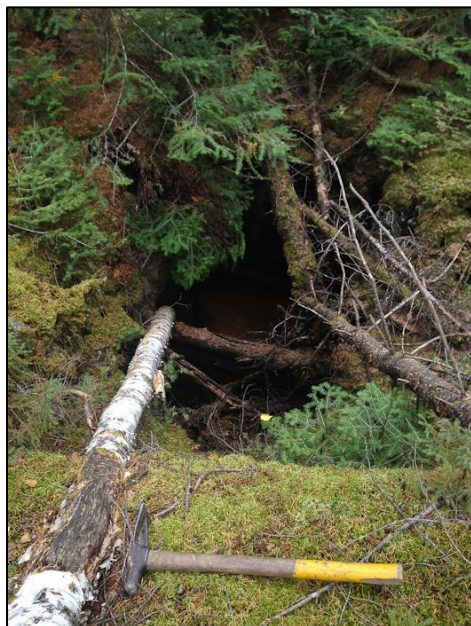
Photos: Kirgood Shaft with steep sides - recommended to fence off hazard (below)
