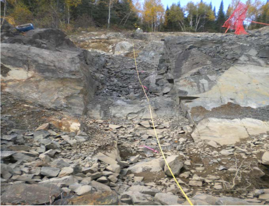
Photo 1 – Trenched and blasted exposure.
