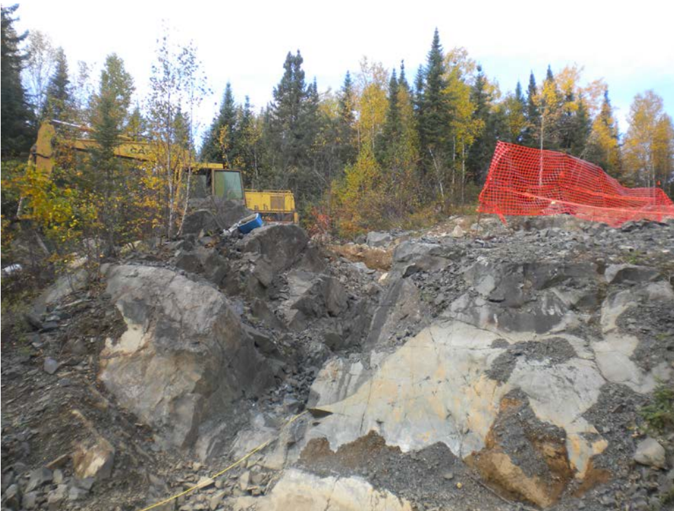
Photo 2 – Blasted pit on edge of outcrop.
