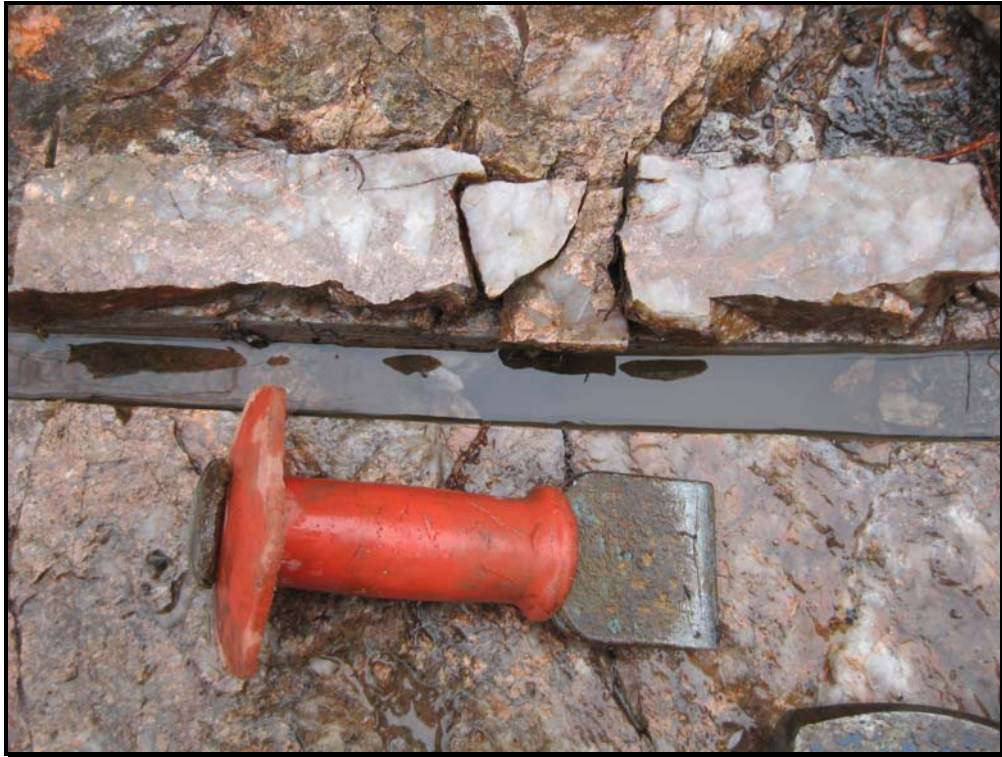
Channel from sample STR13-16 showing shallow vertical extent of quartz and numerous carbonate slips exhibiting movement (chisel pointing west)
