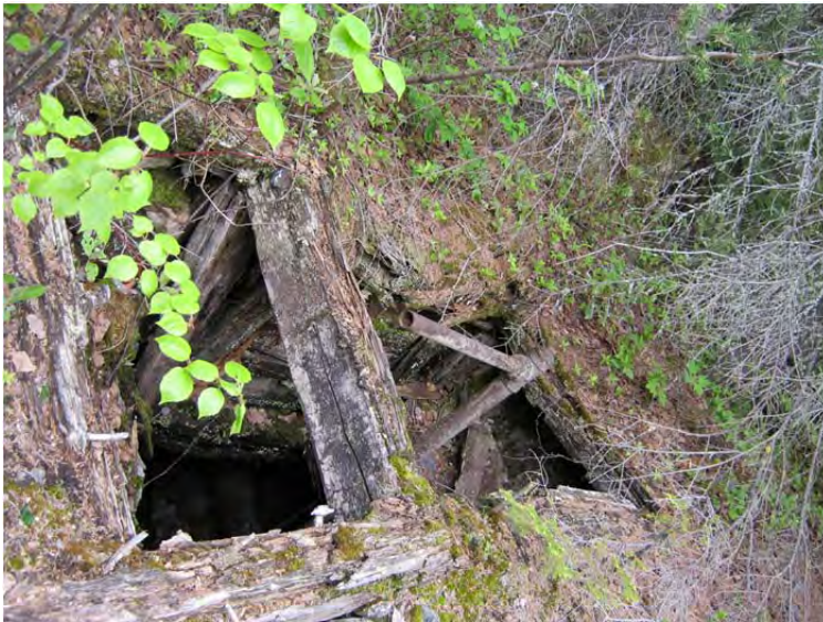
UTM Nad83, ellipsoid height-CENTRE of shaft (2.2m east 70° of point below) (599,116.206E, 5,251,016.26N, ellheight: 265.1)
