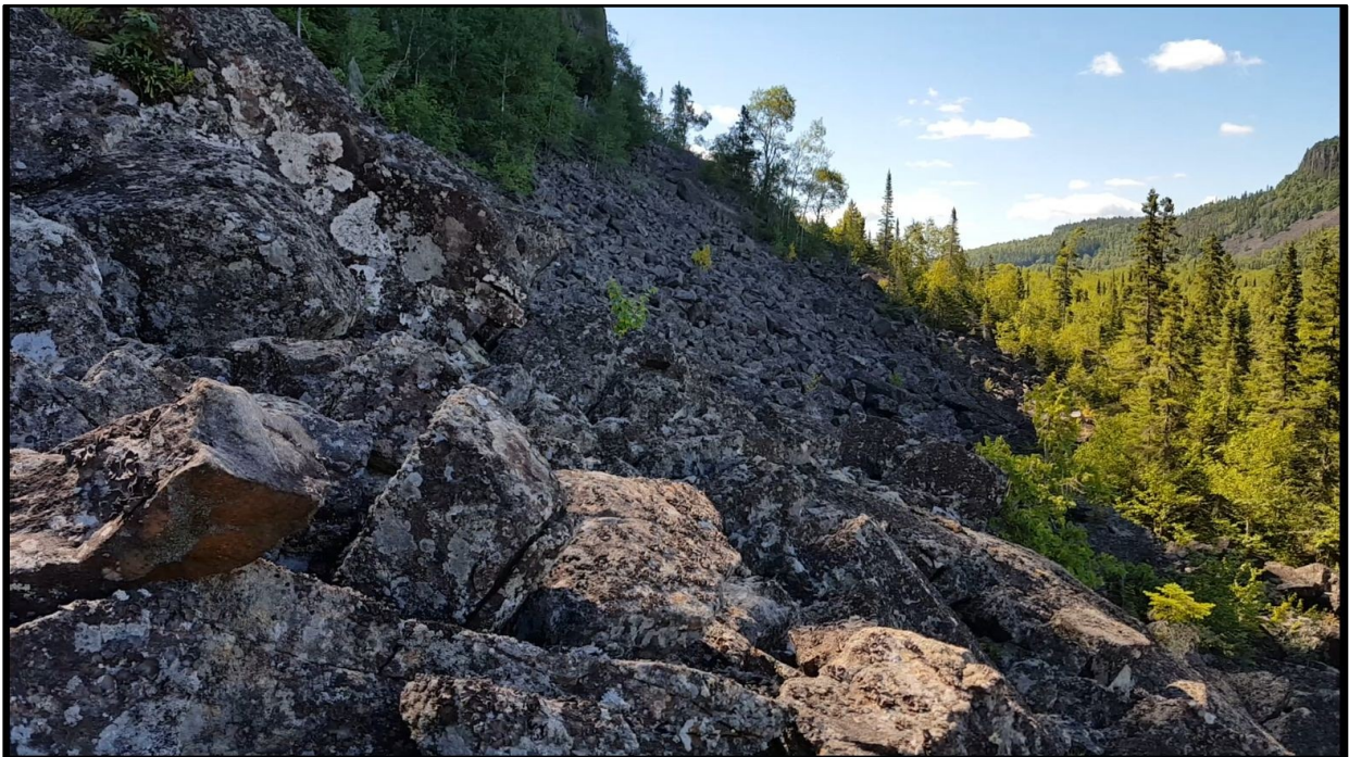
Figure 15: Nature of the talus slope on the east valley wall.
