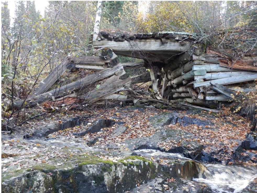
OLD CULVERT ON RIVER
