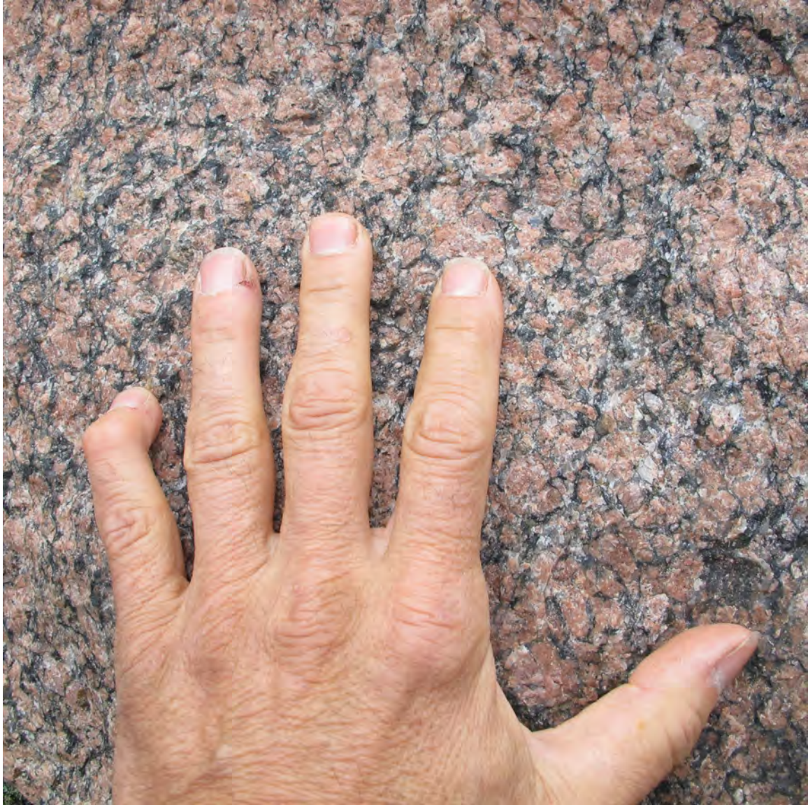
Photo 5: Same area as figure 4 close up showing uniform texture.
