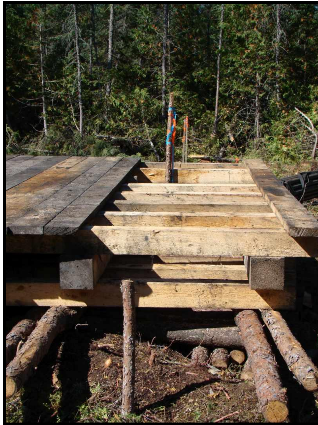
Figure 13: Assembled drill floor with collar and sighting pickets
