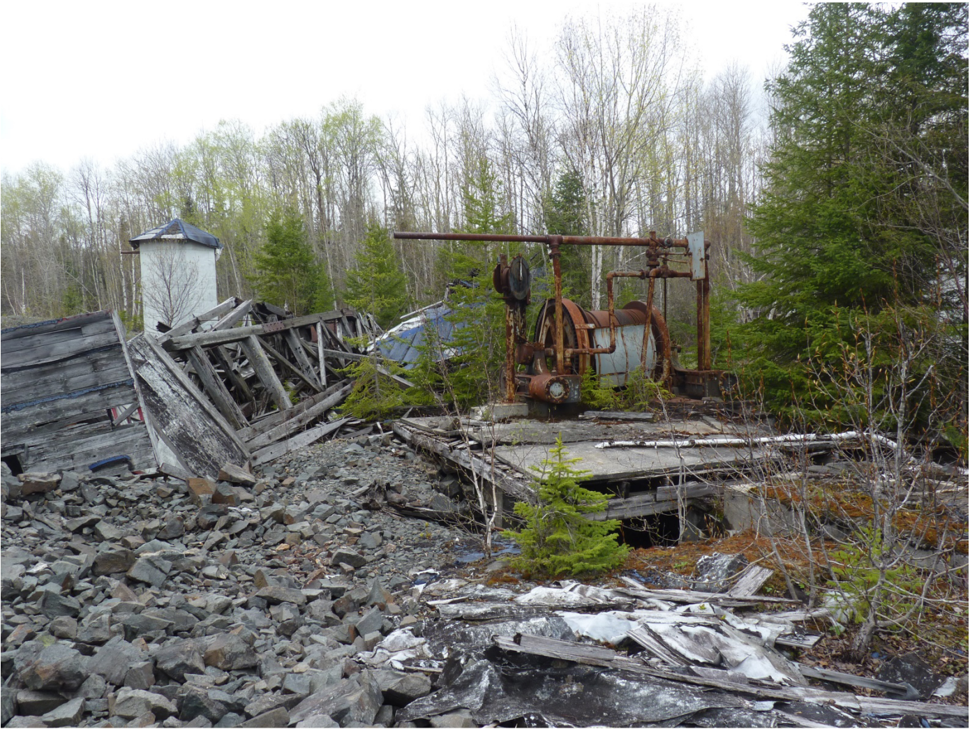
Collapsed Head Frame and Hoist at the Rusty Lake Mine site
