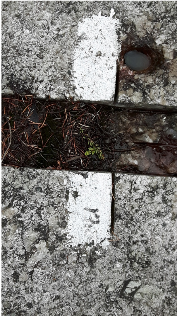
Figure 14-8 Channel SC-01 and a plugger hole on North Dyke
