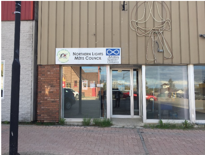
Figure 13-2 Northern Lights Metis Council office in Cochrane
