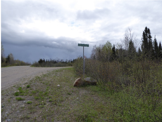
Figure 5-2 Intersection of Translimit Road and Crossover Road
