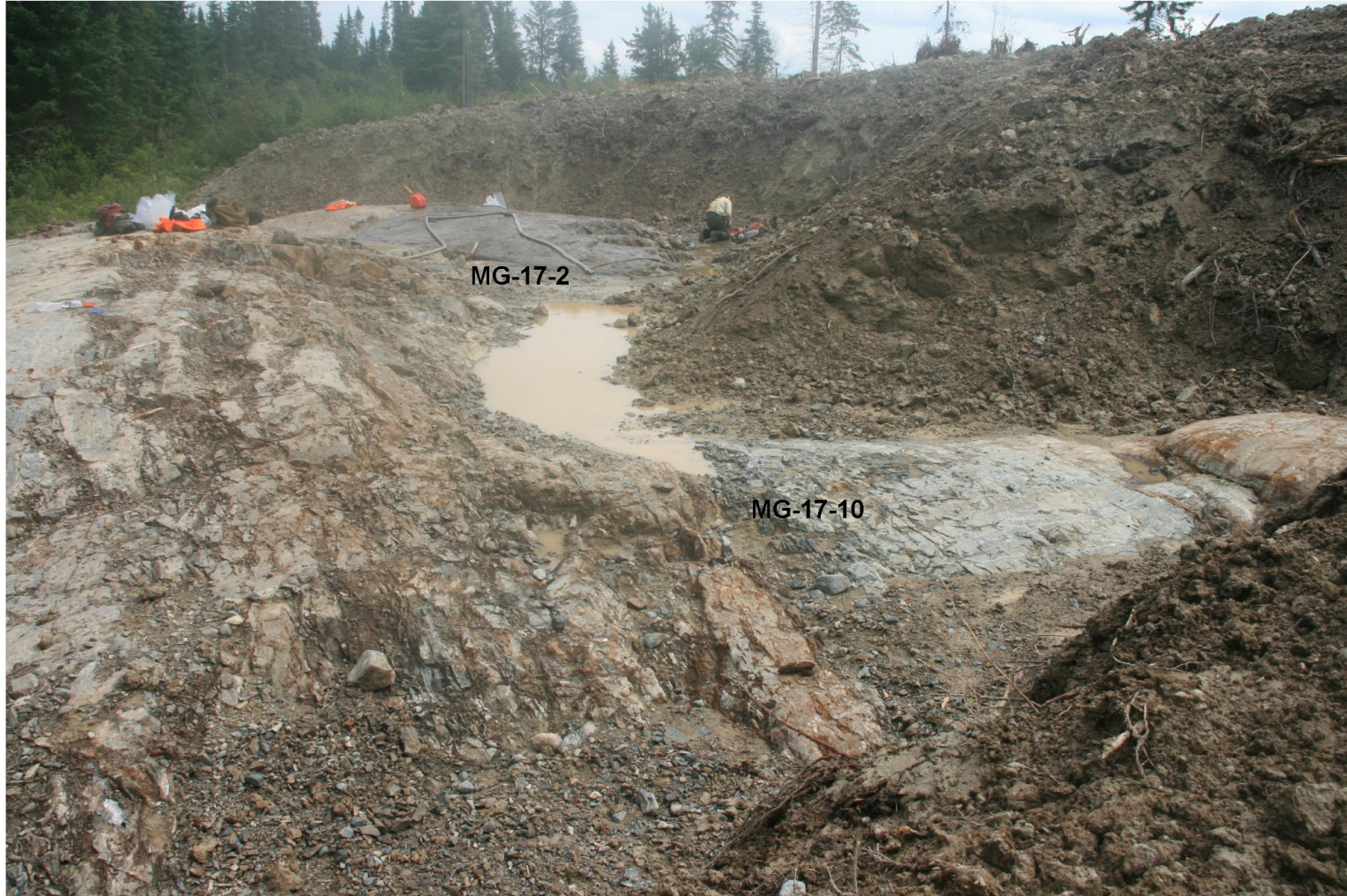
Figure 8: Mugasi Trench, Southwest corner , Channel Cut Locations Tannahill-Holloway Twp., Ontario Looking east
