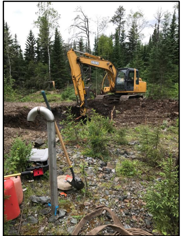
Photo 2 – Excavator by Triumph Shaft Vent
