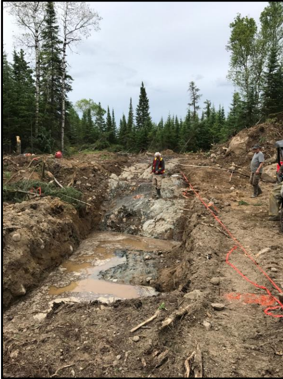
Photo 1 – Ramin on East Shear
