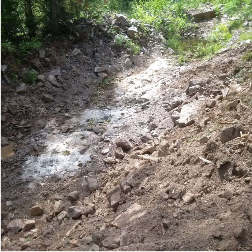
Area 3-b-Mechanical stripping partially complete.
