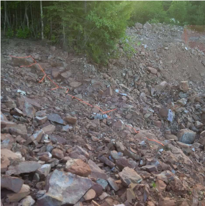
Area 1-b Ready to blast new trench
