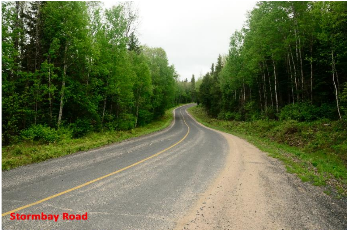
Figure 5.1 Photos showing the general condition of roads used to access the Black Jack Project area.
