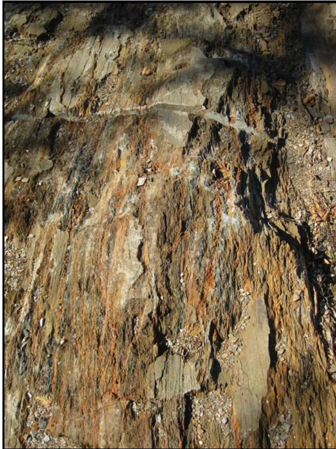
Plate 1: deformation zone on Flint Block typical of the area
