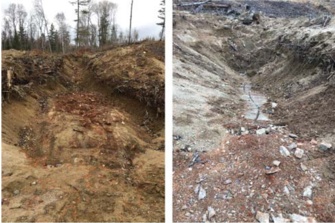
Figure 10. Trench G looking north (left) and west (right)
