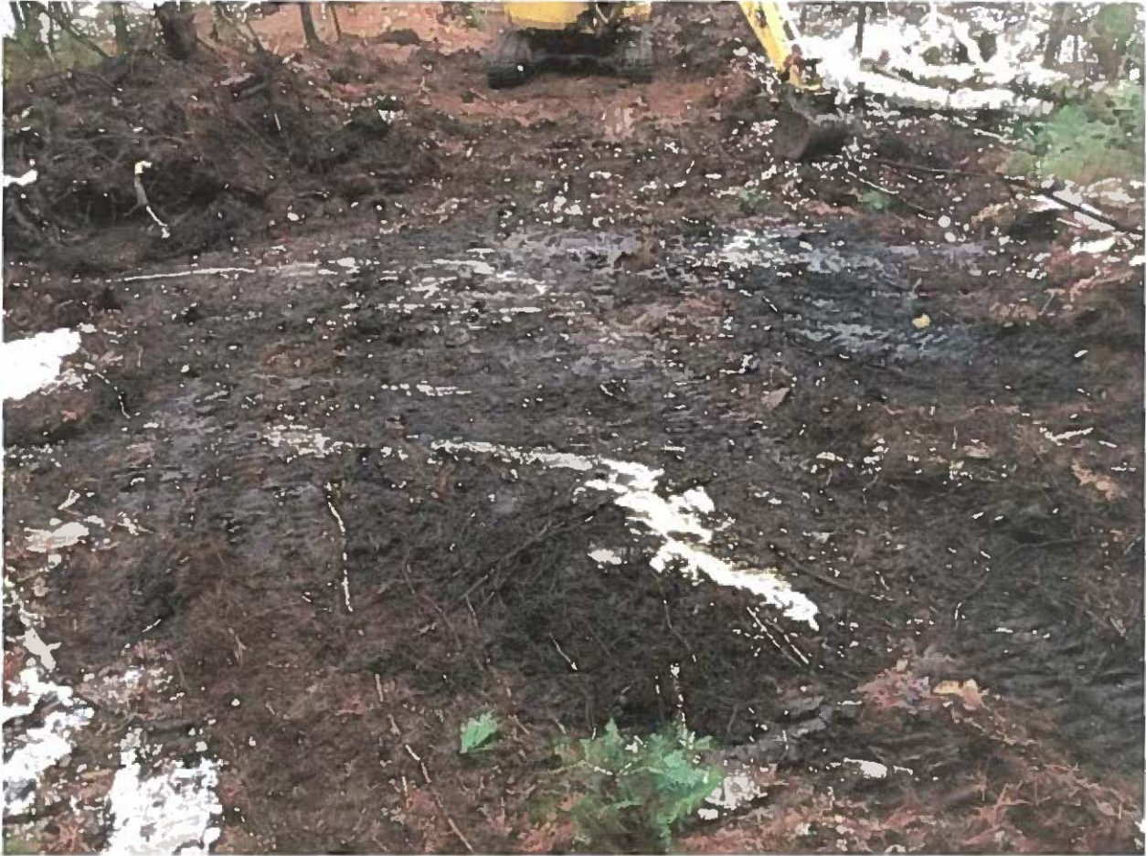
Picture 3: Clearing of Area 2
