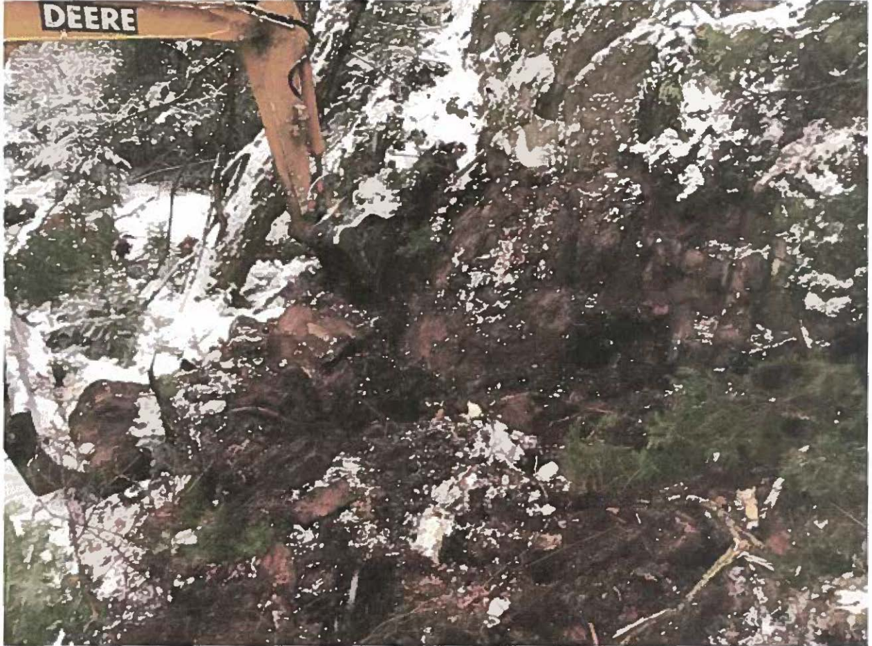
Picture 4: Stripping of Area 1
