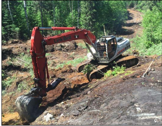
Figure 9: Excavator working beside a rare natural outcrop
