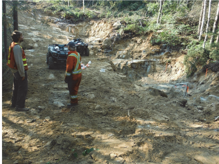
Figure 23 – Photo of Trench 31W
