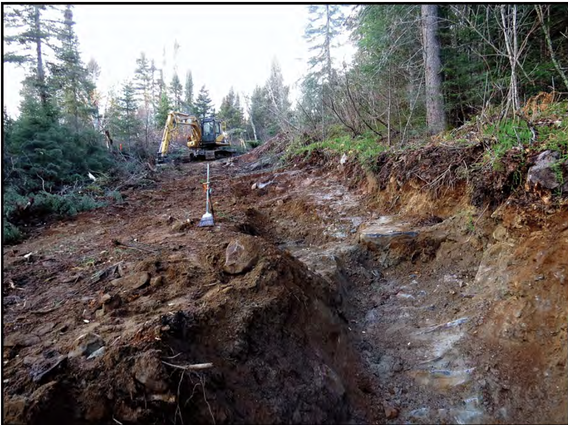
Figure 7: Strip 2 and excavator
