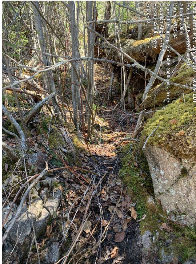
Figure 6: Overgrown Baker West Trench
