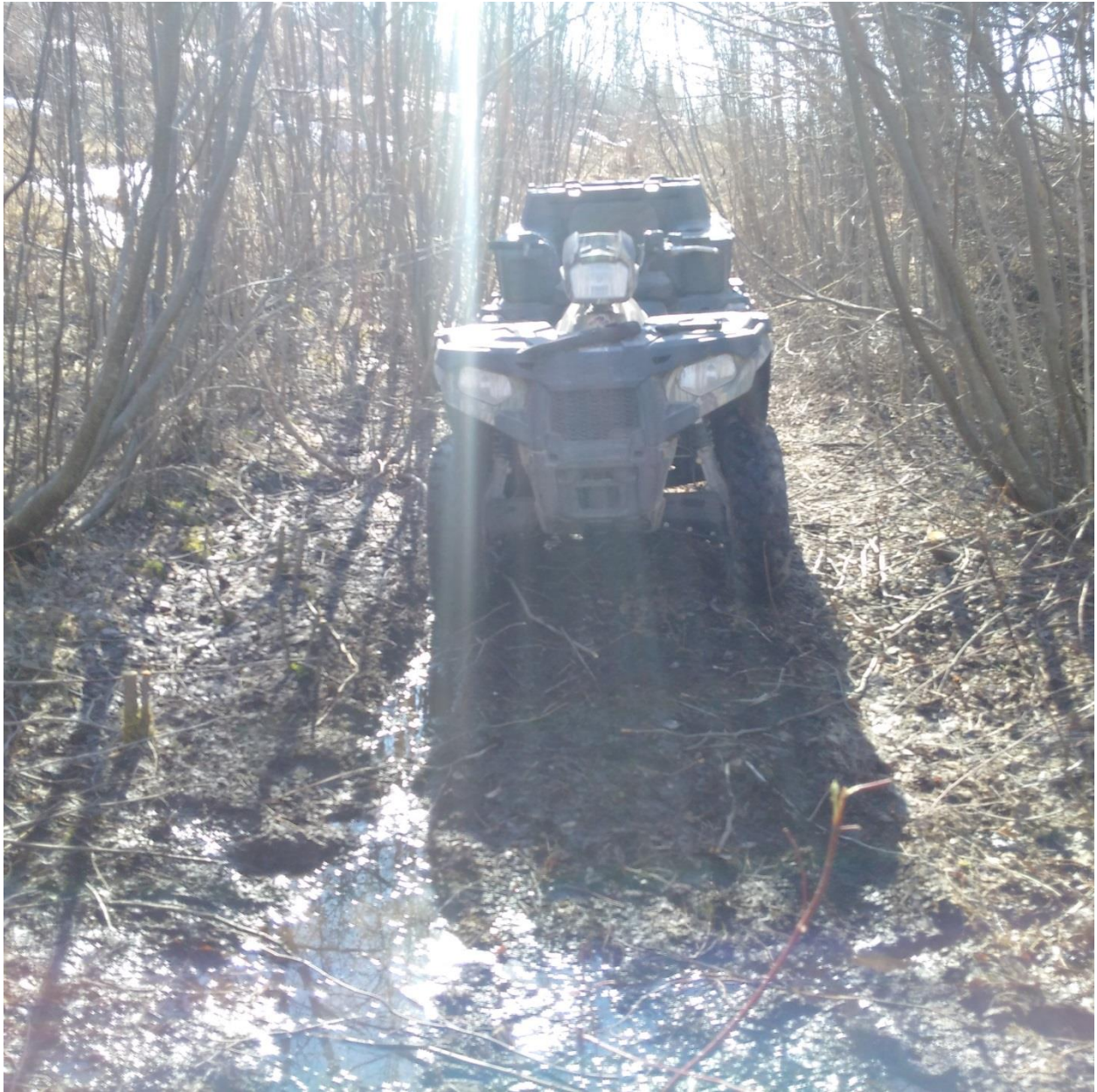
Figure 12 – Trail Clearing for 2020 Drill Season (Start of Trail)
