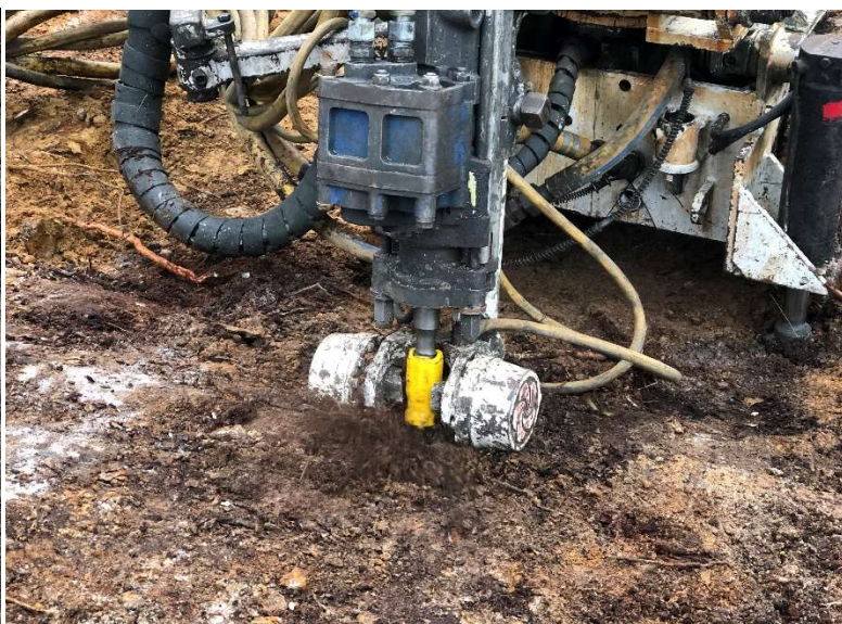
percussion drill set-up
