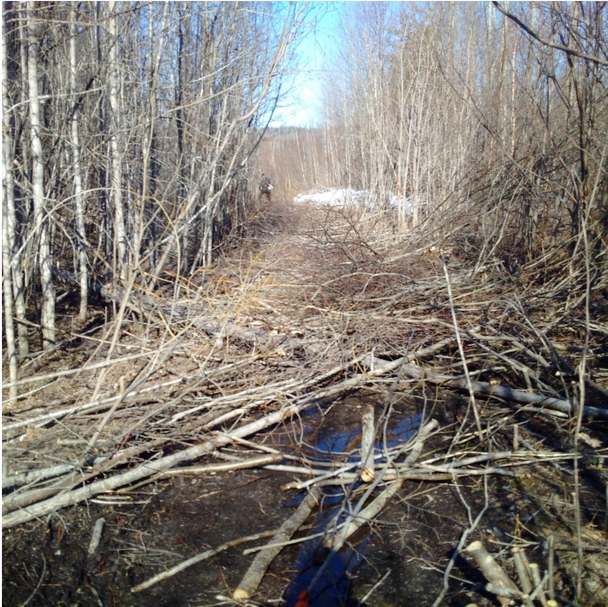
Figure 5 - Initial Trail Clearing
