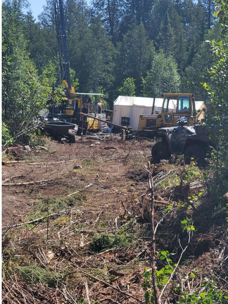
Figure 12 - Drill Hole 2 Setup
