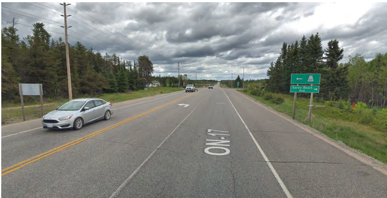
Figure 5-1 Turn off Highway 17 onto Highway 601.
