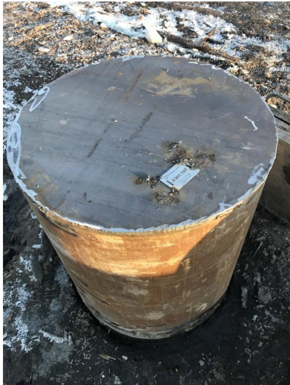
Figure 14: Clean drill site with capped casing and well tag (Z19-4FM08)
