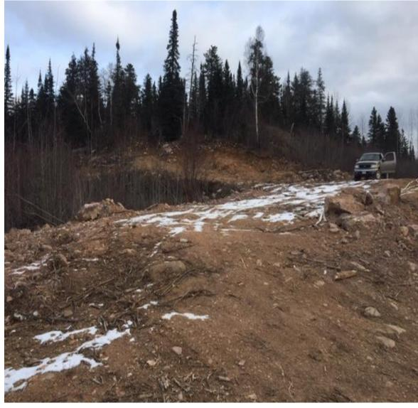
October 19<sup>th</sup> area stripped ,removed overburden large rocks. Looking west from granite out crop. Large rocks used as buffer wall to right of photo. Far back of photo area excavated and stripped dates of November 26,27<sup>th</sup>.
