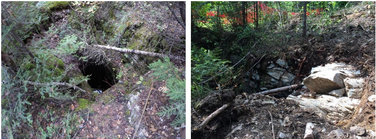
Figure 5. Photos of upper Sunbeam shaft before (left) and after (right) stripping
