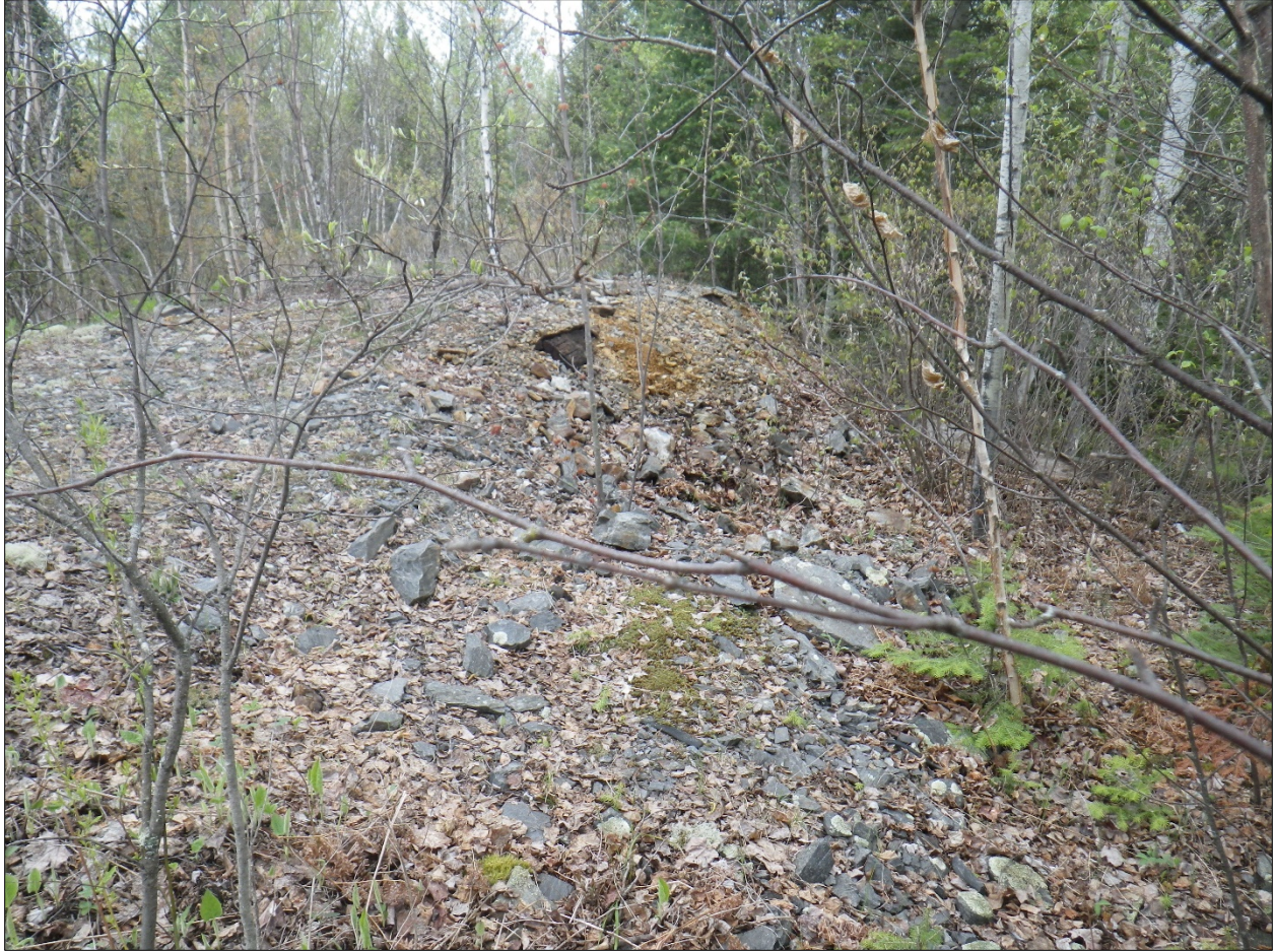
Figure 6: Cribbed rusty muck pile adjacent possible Ludwig test mill site.
