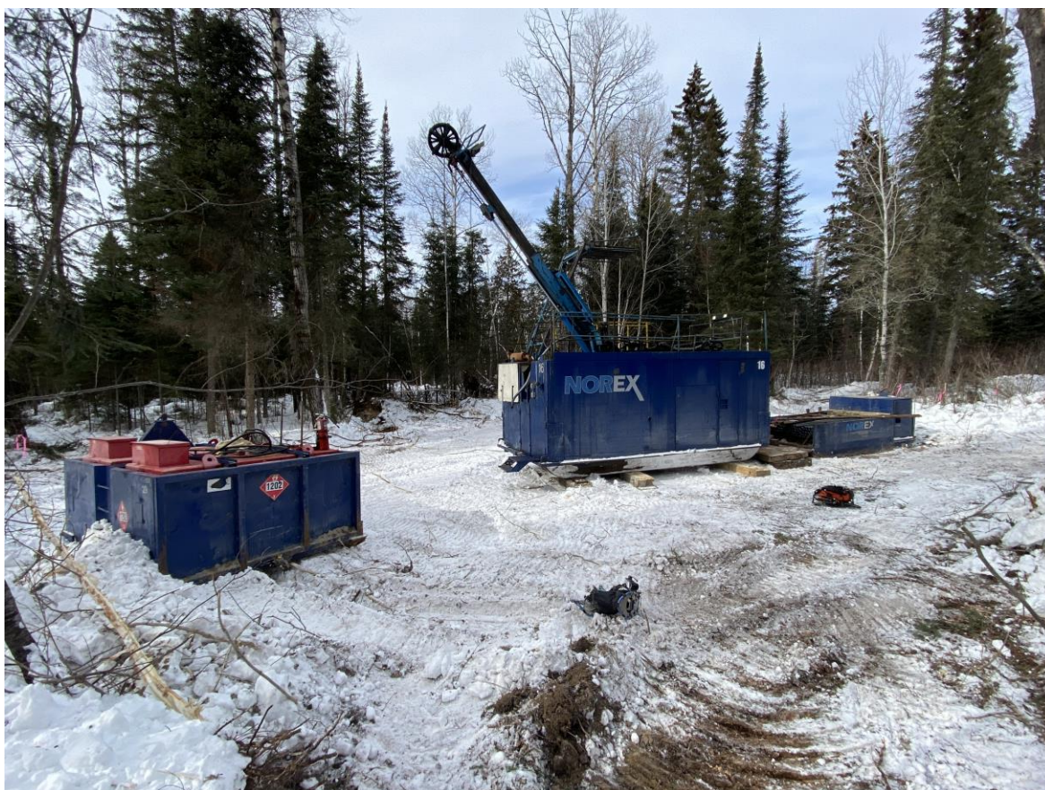
Photo 1 Drill rig at GP20-01 site
